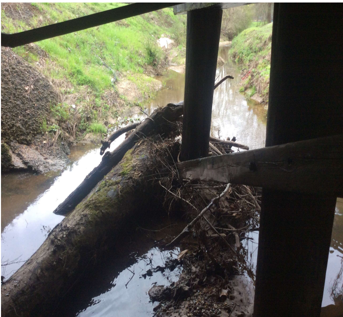
PHOTO 1 Description Bent 2 drift right side, against Pile 4.
