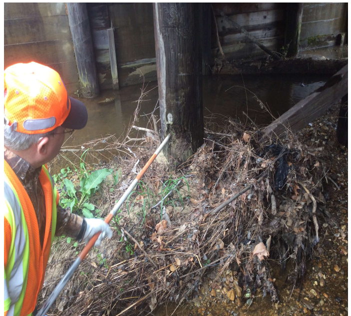
PHOTO 2 Description Bent 2 pile 1 rotten
